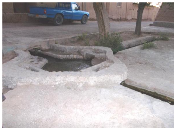
Fig. 2: Qanat water channel entering the village, Yazd province, Iran (Photo by: Michaela Ibrion, 2012).
