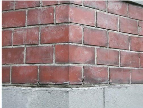
Fig. 1: Red brick-like tile used for the façade of the Governor General Building, Taipei, Taiwan.
