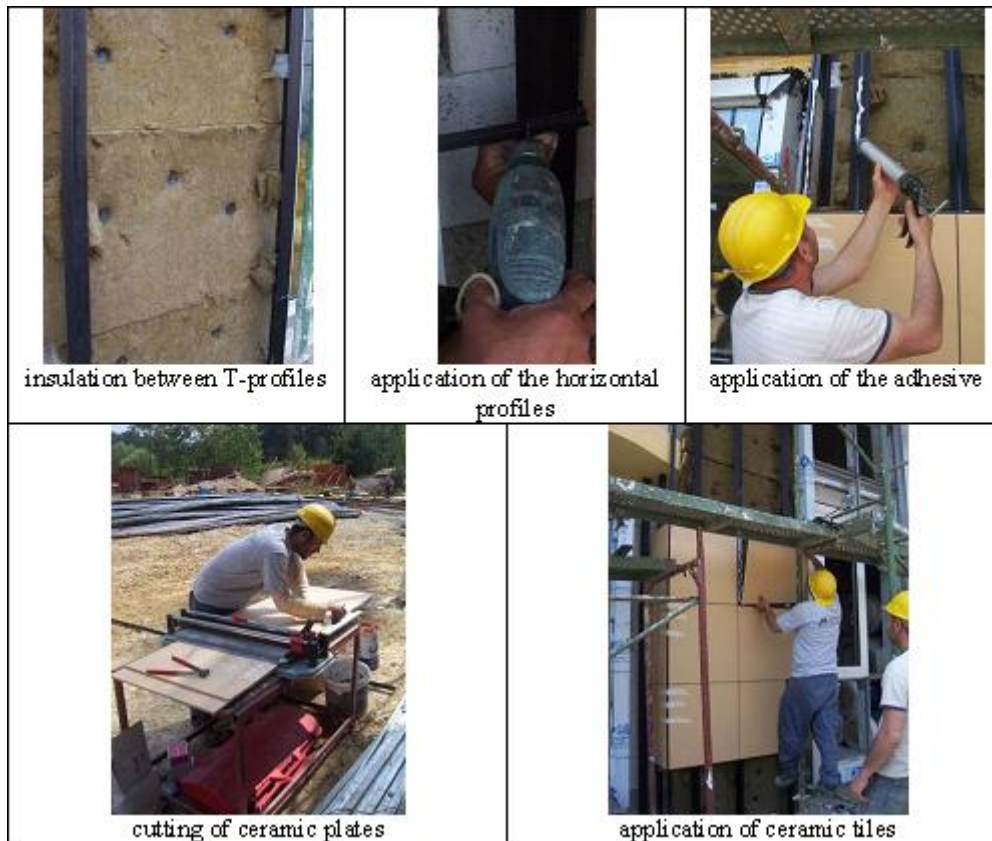
Figure 2. Steps of construction.
